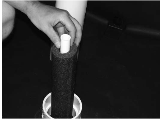
Step 8 Slide the pipe insulation on the 3/4" fill line. Leave it about 1 1/2" down from the top of the pipe.
