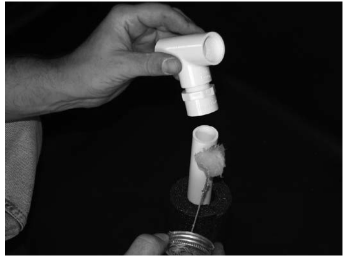
Step 10 After the fitting is tightened into the "T" fitting, apply PVC cement to the 3/4" pipe and install the "T" assembly.
