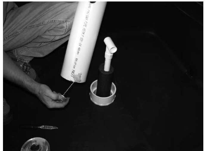
Step 12 Apply PVC cement to the bottom of your 4" pipe.
