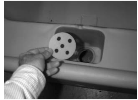
Step 9 Insert the poly drain screen in the overflow hole to keep unwanted debris out of the system for constant flow only, otherwise place a 3" rubber drain plug in this opening.
